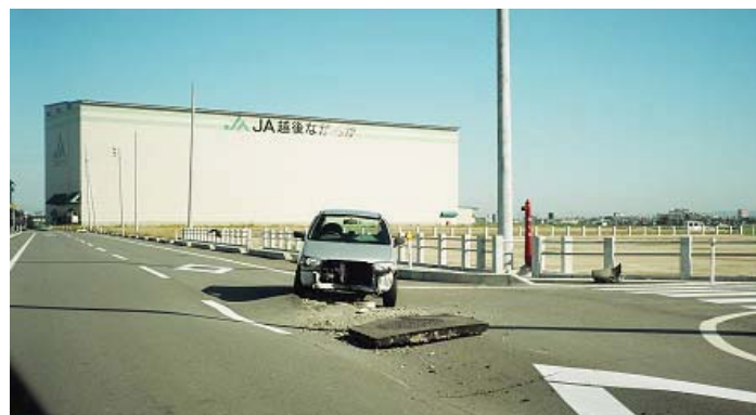
Fig. 5.2 Car collided with uplifted manhole in Nagaoka city after the 2004 Niigata-ken Chuetsu earthquake, Japan (Technical Committee on the Sewer Earthquake Countermeasures, 2005).
