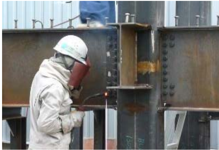
Figure 5.4 Vertical welding in web
