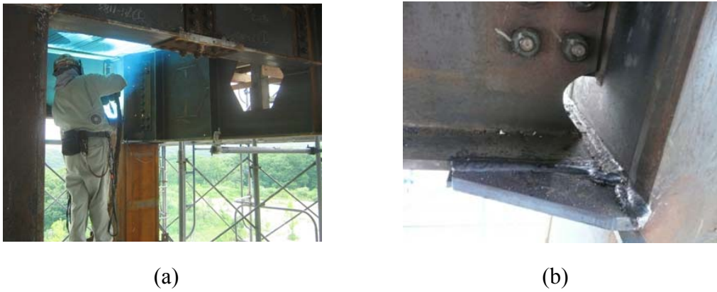
Figure 6.8 Wing plate connection: (a) Welding situation; (b) Close-up view
