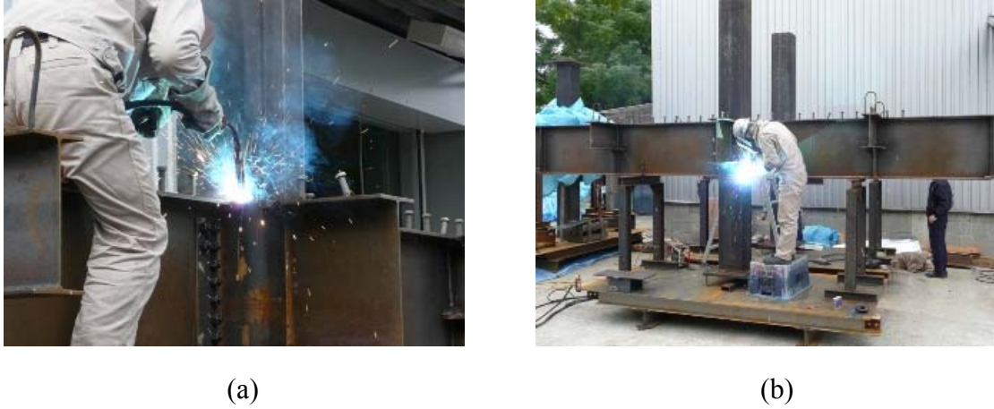
Figure 5.3 Field weld situation: (a) Top flange; (b) Bottom flange
