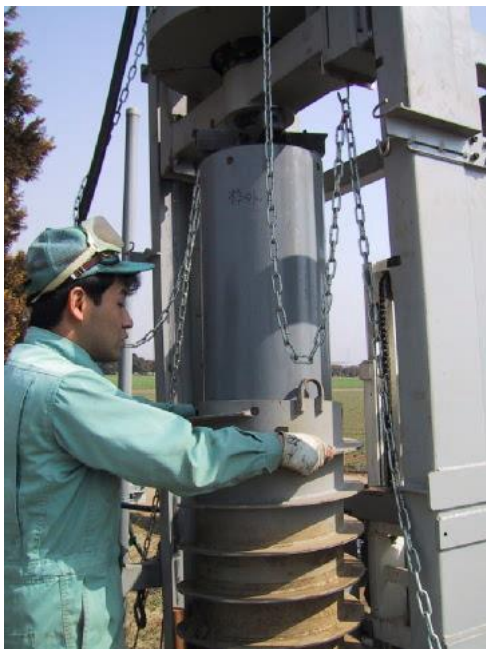
c) Install the drill cylinder outside the PVC casing
