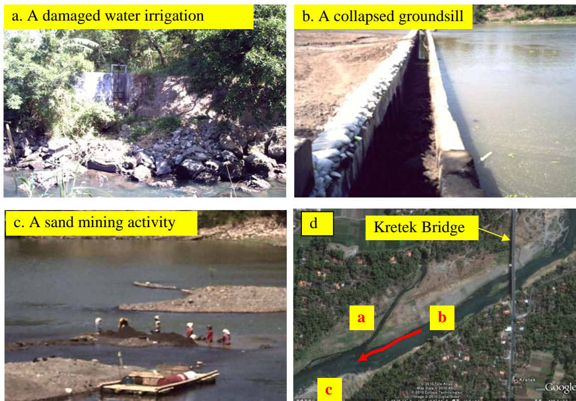
Photo 2.6 Impacts of riverbed degradation due to sand mining activity in the downstream of Opak River. Photos a, b, c were taken in June 2007 (Figure d source from Google Earth, 2010)
