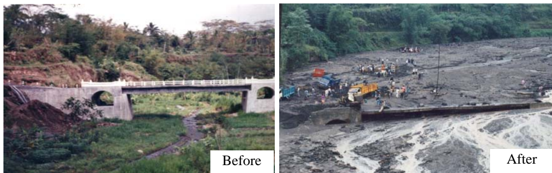
Photo 1.2 Kemiri Bridge on Boyong River after a debris flow in 1994 (Photo courtesy Adhy Kurniawan)
