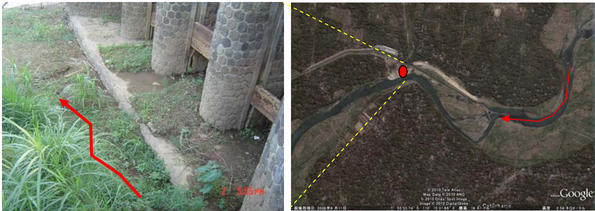
Photo 2.5 The Saphon irrigation intake. The photo shows the water can not enter to the irrigation intake due to severe bed degradation (Photo courtesy Masaharu Fujita)
