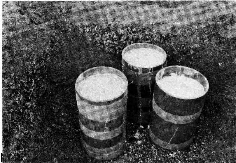
Photo 9.2 Block sample covered with a tube of vinyl chloride
