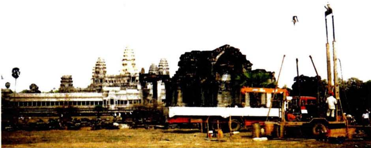
Photo 3-1 The first deep boring at Angkor Wat
