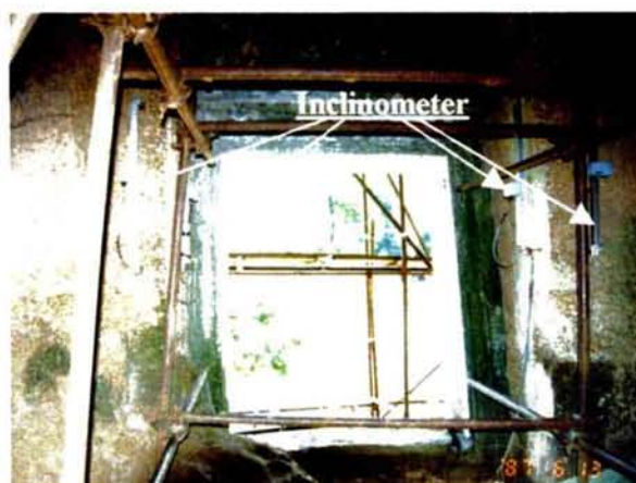
Photo 6-13 Vertical inclinometer installed at walls inside N1 Tower, Prasat Suor Prat
