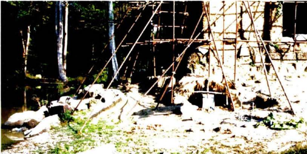
Photo 6-14 Settlement Gages at N1 Tower, Prasat Suor Prat
