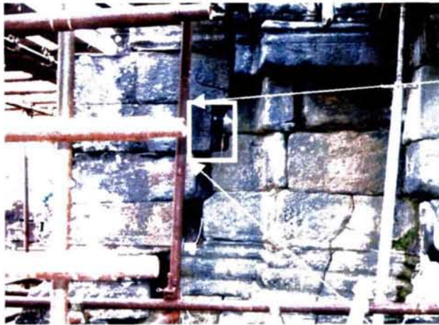
Photo 8-9 Gap gage to measure change of vertical opening between stone elements
