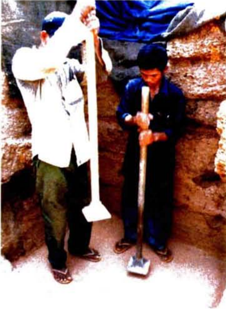
Photo 8-14 Manual compaction using "elephant foot".
