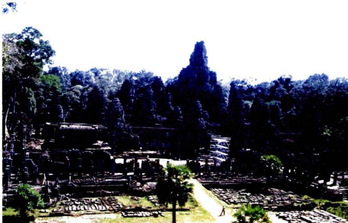
Photo 8-19 Arial view after completion of restoration of North Library from north.
