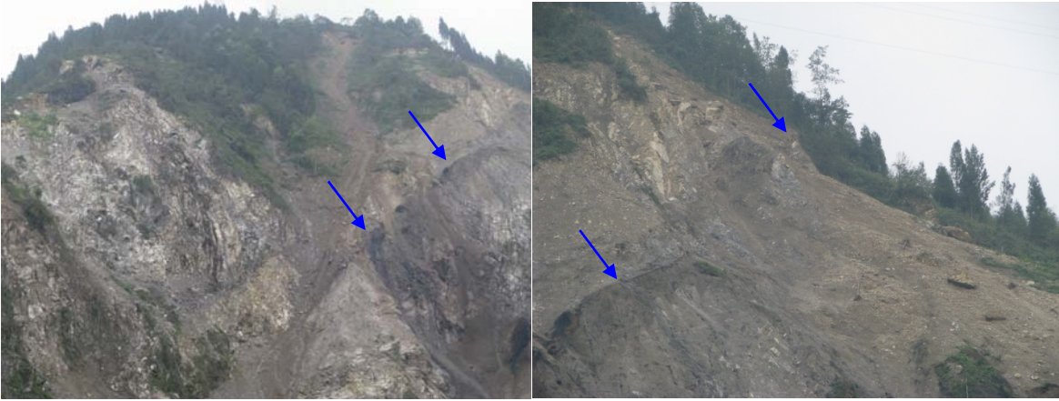
No.5. Qingping. Top: Looking to NW. The fault runs beyond the two persons, then crosses the river with a small fall, then climbs up to the cliff in the right. Lower left: The fault is indicated by arrows. Lower right: On the right of the lower left figure; the surface is displaced with thrust up of the left side.
