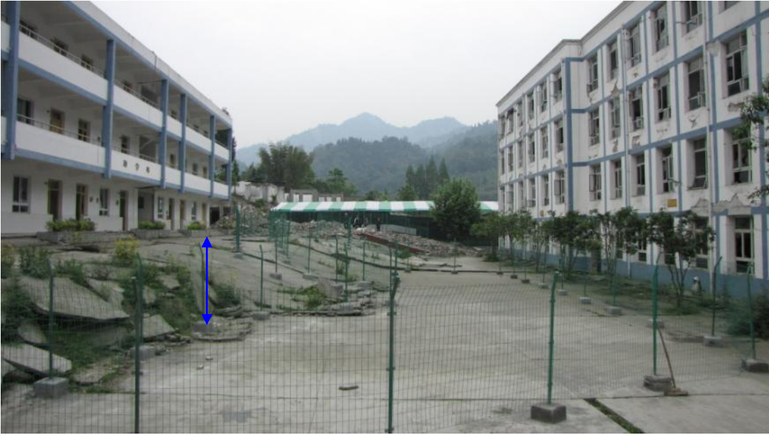
No.12 Bailu (Looking NE). Left side upheaved 2 m.
