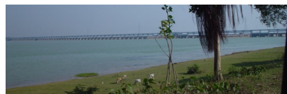
Photo.3 Farakka barrage in India
