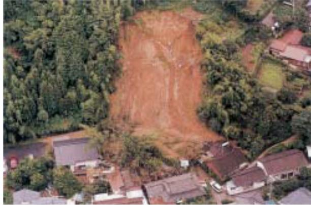
Figure 1.7 Slope failure due to torrential rainfall of the Bai-u front (Minamata City, Kumamoto Prefecture, July 1997) (*Photo Courtesy: MLIT, Japan*)
