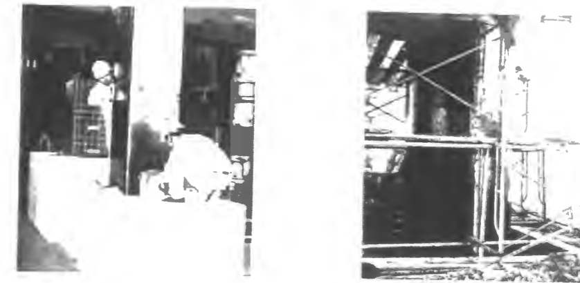
Figure 2.17 FRP wrapping method
