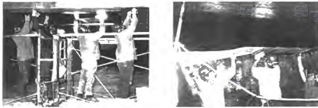
Figure 2.4 CFS retrofitting for flexure
