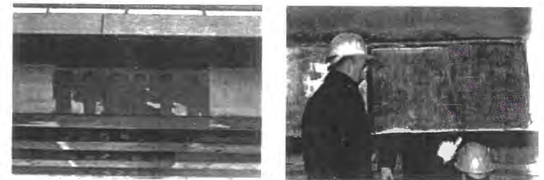
Figure 2.6 FRP retrofitting for shear
