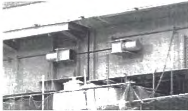
Figure 2.21 Cable restrainer for superstructure movement joint
