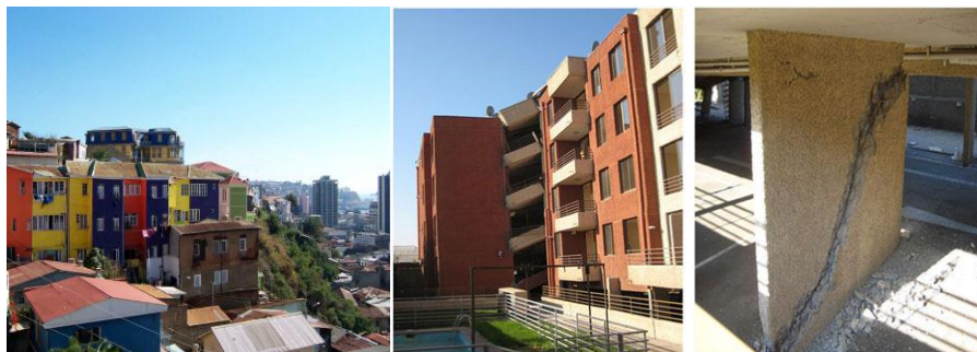
Figure 2.18 Adjacent buildings in a crowded city
