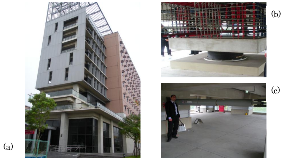
Figure 6.20 (a) Civil engineering research building of the National Taiwan University (b) Lead rubber bearing (c) Viscous damper
