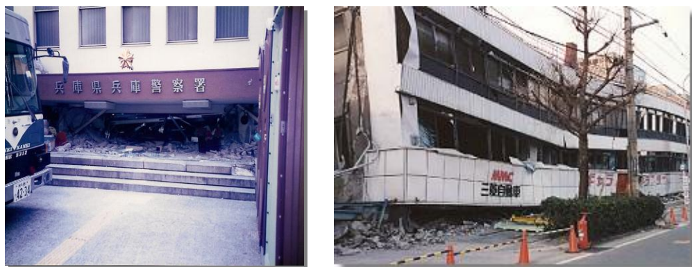
Figure 6.3 Soft story failure (Kobe earthquake, January 17, 1995, magnitude 6.9)
