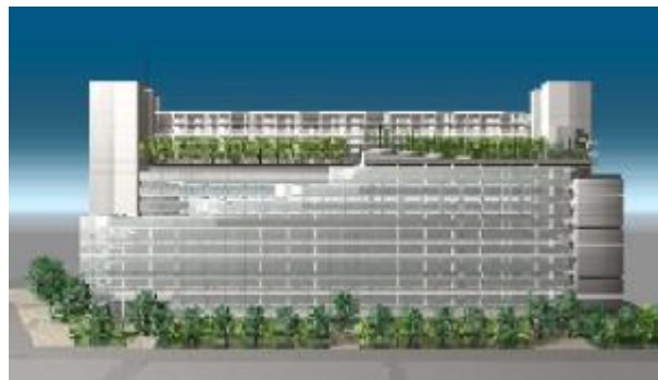
Figure 6.17 External view of the building constructed with mid-story seismic isolation (Murakami et al 2000)
