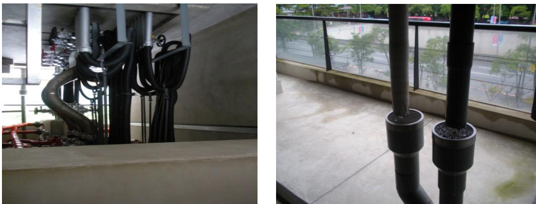
Figure 6.21 Non-structural components at the seismic isolation level
