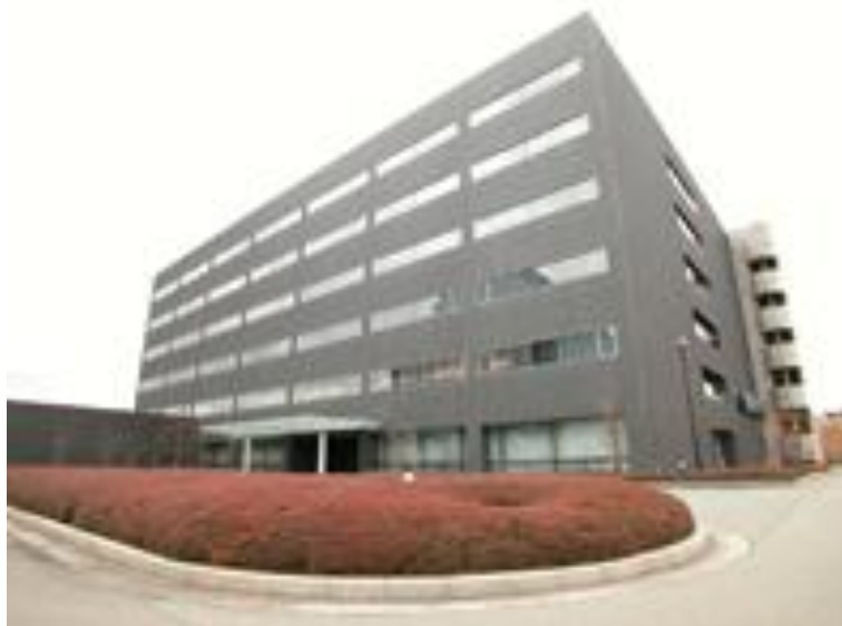
Figure 1.7 West Japan Postal Savings Computer Centre in Sanda, Kobe, Japan
