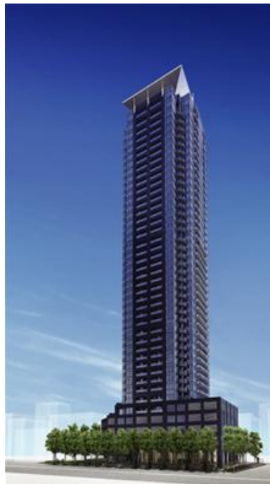
Figure 1.9 43-story high rise condominium base isolated building, Japan [12]
