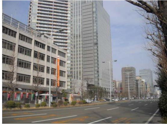
Figure 1.8 29-story base isolated reinforced concrete building survived during 2011 Tohoku earthquake, Japan without structural damage
