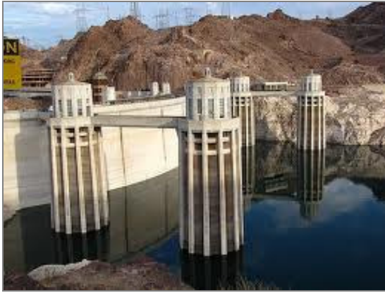
Fig 2.1 Water source intake (myalucardster, 2011)
