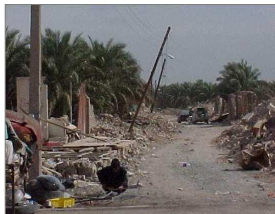
Fig 2.19 Collapse of the buildings
