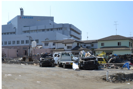
Photo 23 Remained houses behind RC building
