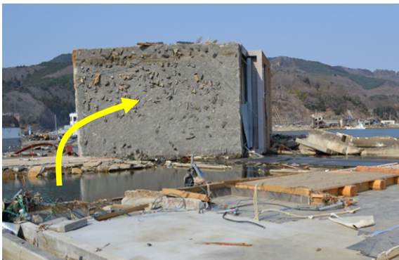
Photo 45 Toppled RC 3-story building
