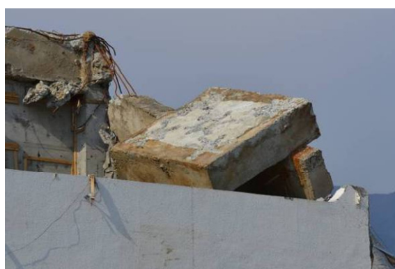
Photo 6 Pile cap of building C
