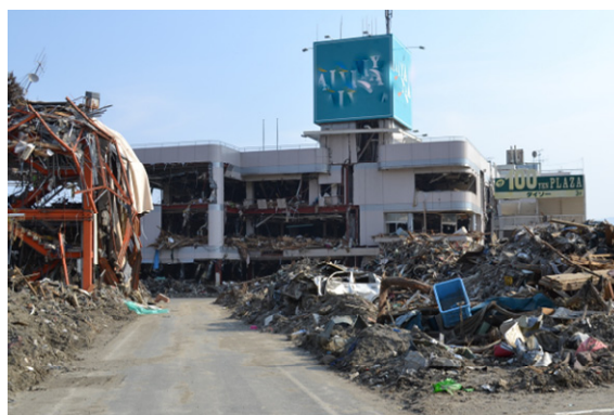
Photo 10 Building D (Mountain side)
