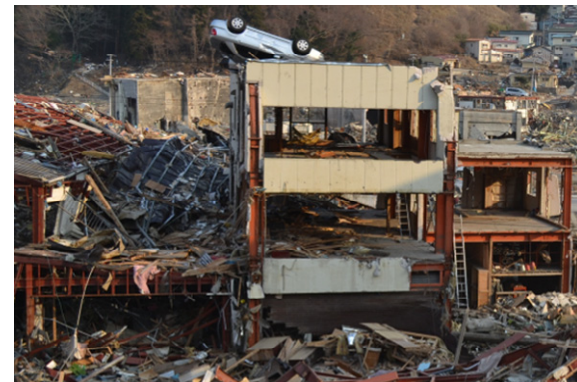
Photo 30 Car on steel 3-story building
