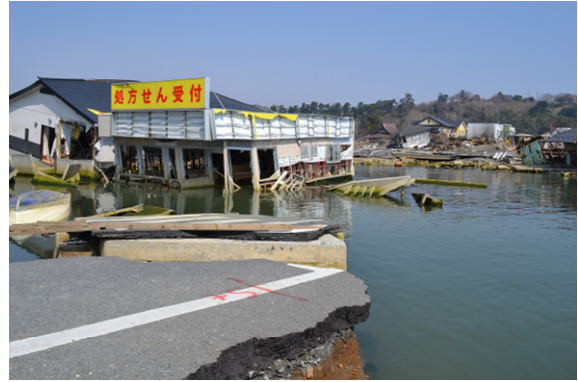
Photo 22 Road washed away by tsunami (Ishinomaki-city)
