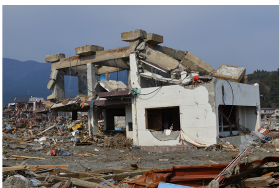
Photo 5 Overturned building C
