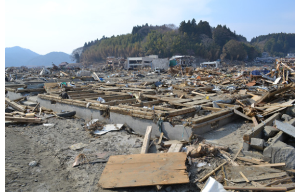
Photo 14 Remained house's foundation
