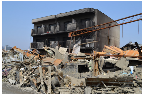
Photo 18 RC 3-story building, damage caused by Tsunami and fire
