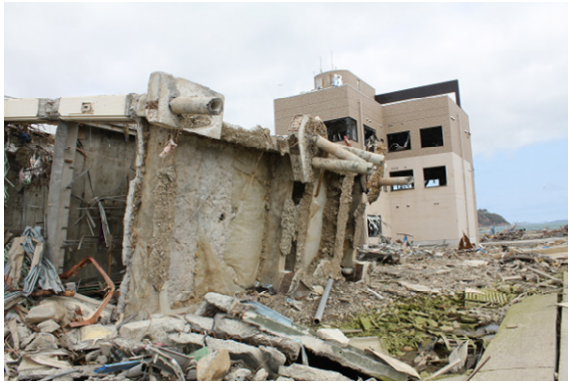
Photo 41 Toppled building H
