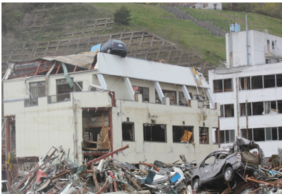
Photo 31 Car on RC 3-story building
