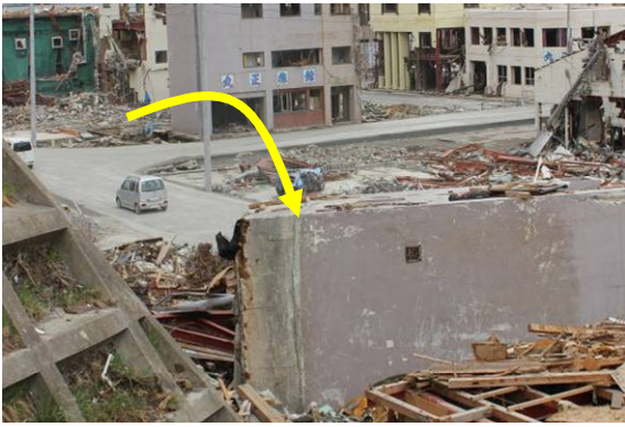
Photo 33 RC building E carried 70 m away and toppled
