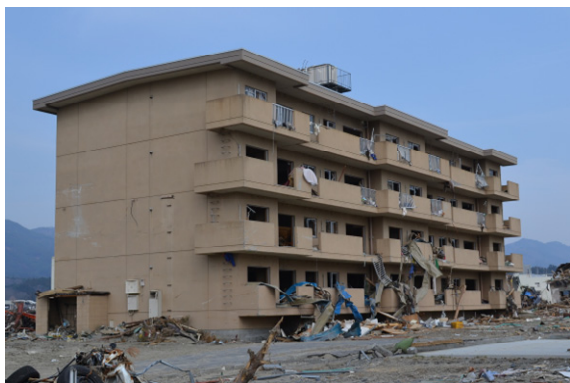
Photo 3 RC 4-story building B, tsunami reached 4th floor
