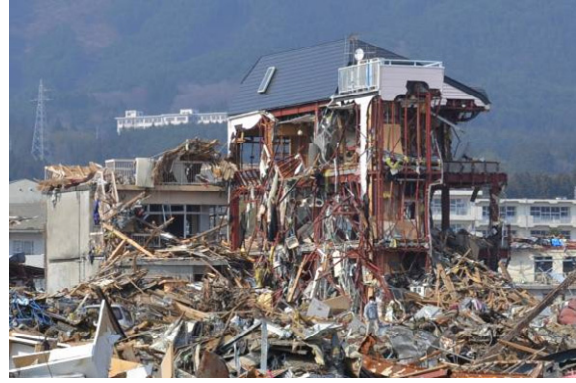
Photo 12 Damage to steel structure
