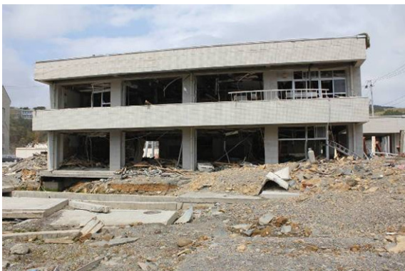
Photo 47 Building J at sea-side
