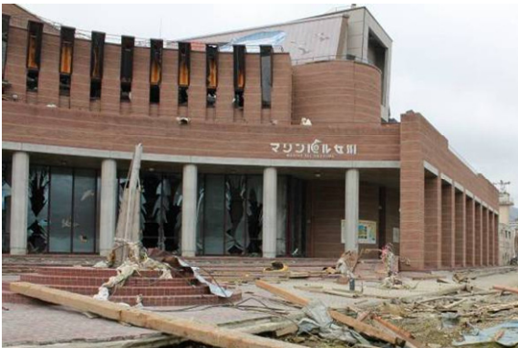
Photo 43 RC 3-story building I at sea-side
