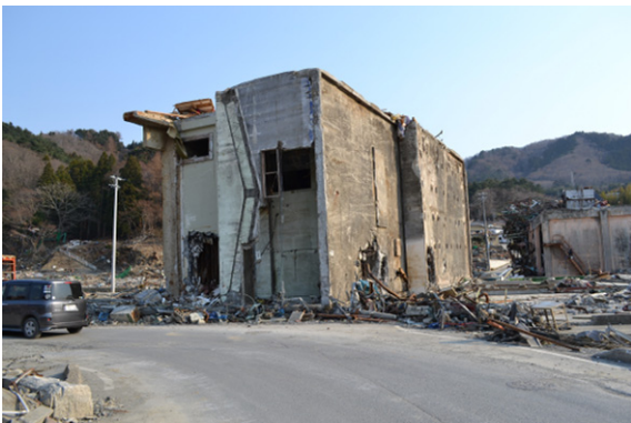
Photo 39 Toppled RC 2-story building G
