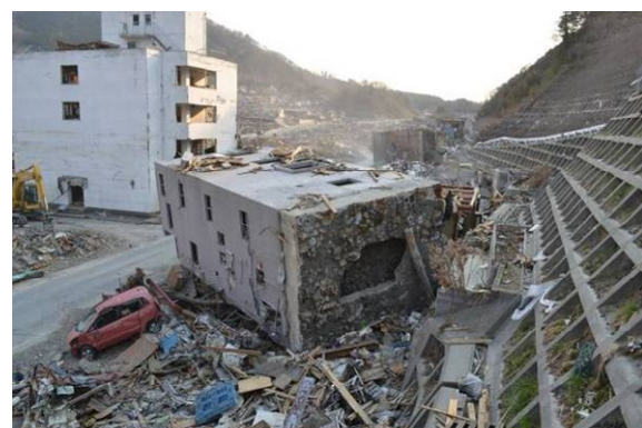
Photo 32 Topped RC 4-story building E
