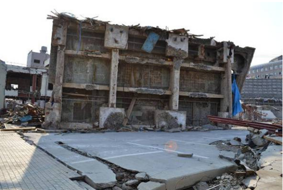
Photo 37 Toppled building F
