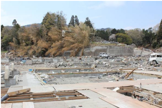
Photo 53 Remained house's foundation
