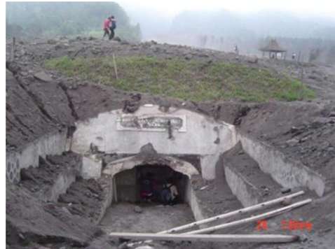
Photo 1 Bunker buried by the pyroclastic flow 2006 where two people were dead
