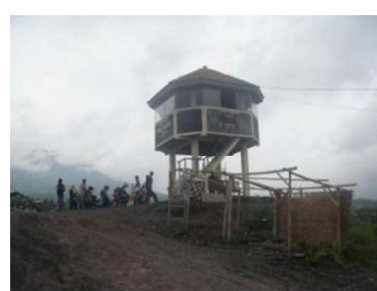
Photo 12 Monitoring tower by NGO in Gendol River
