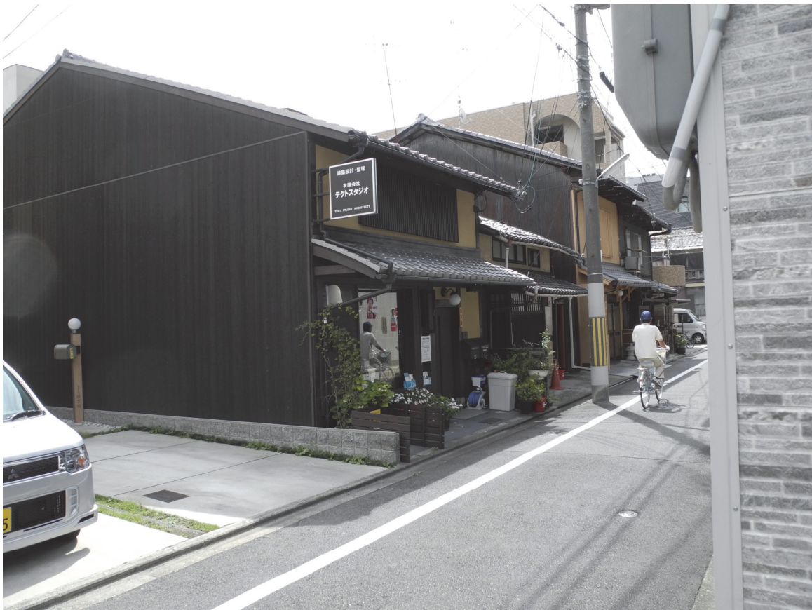
Fig. 6- 20 House corresponding to case 5 seen from the outside.
