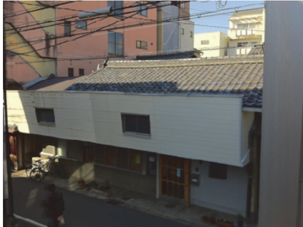
Fig. 7- 4 Same building in a different angle.
