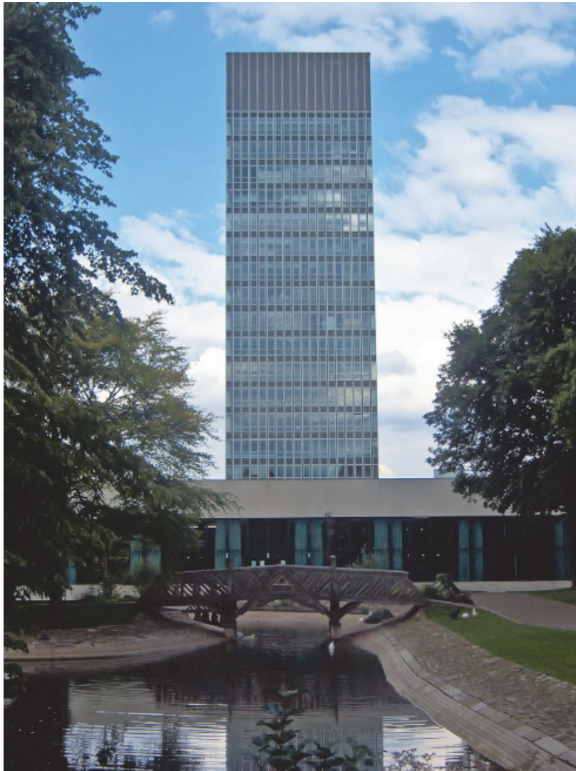
Fig. 2- 7 Sheffield University designed by Gollins, Melvin, Wards and partners. Source: (Wikipedia, 2010)
