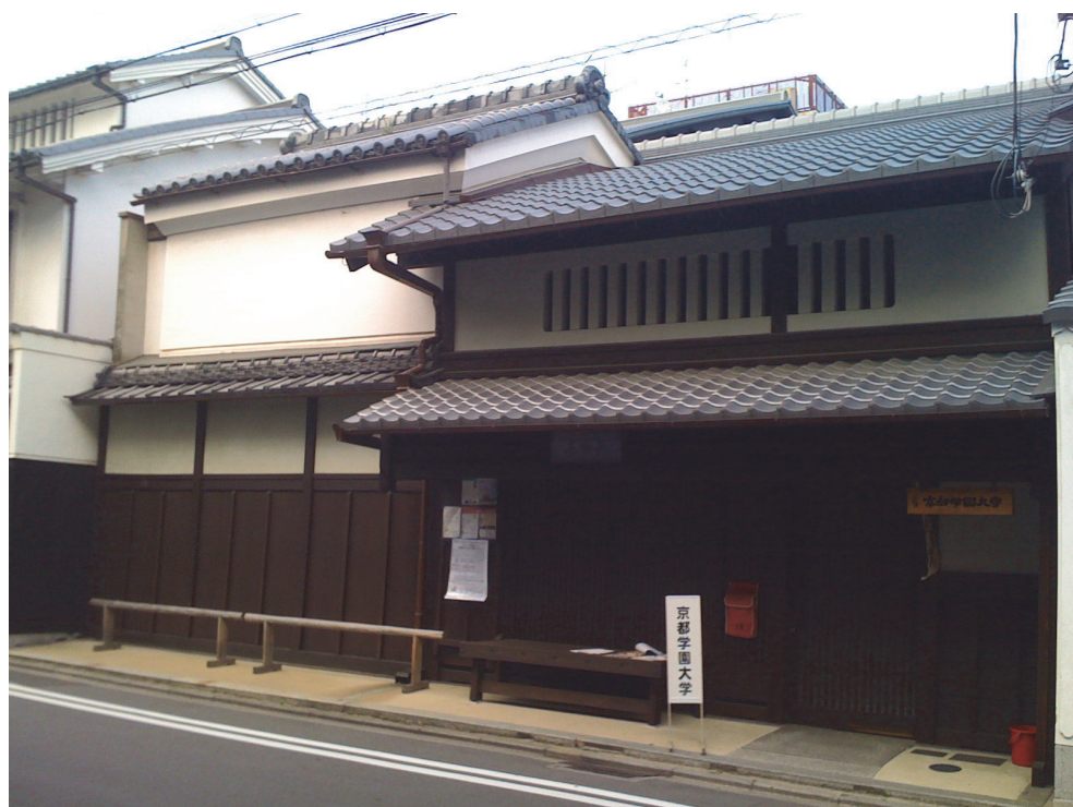
Fig. 6- 1 Façade of building corresponding to case 67.
