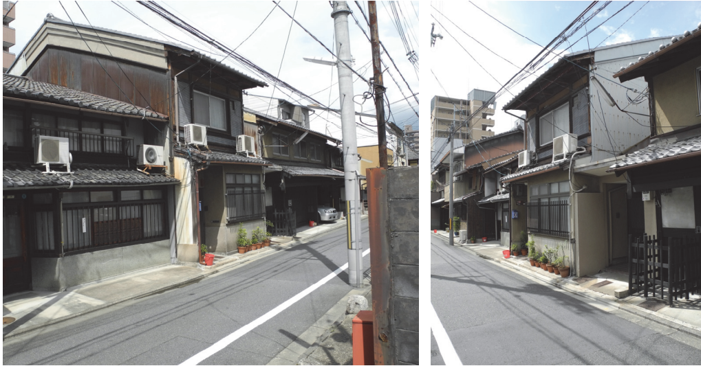
Fig. 6- 24 House corresponding to case 6 seen from the outside.
