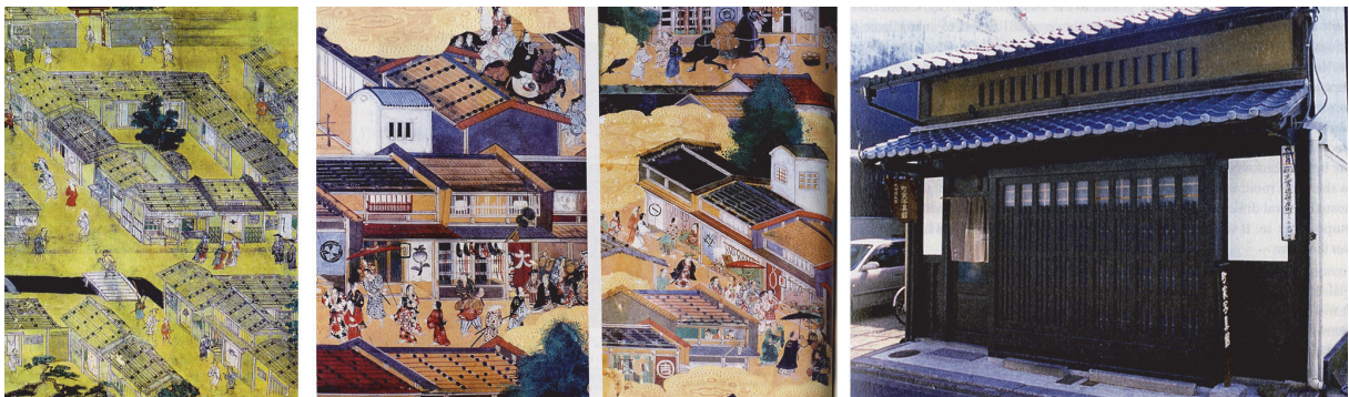
Fig. 1- 2 Sequence of images showing evolution of Machiya. From left to right: Fragment of "Machida-bon" 16th century, two fragment of "Ikeda-bon" from the 17th century, A Machiya as still can be seen in Kyoto. Source: Machiya, architecture and history of the Kyoto town house (Löfgren, 2003).
