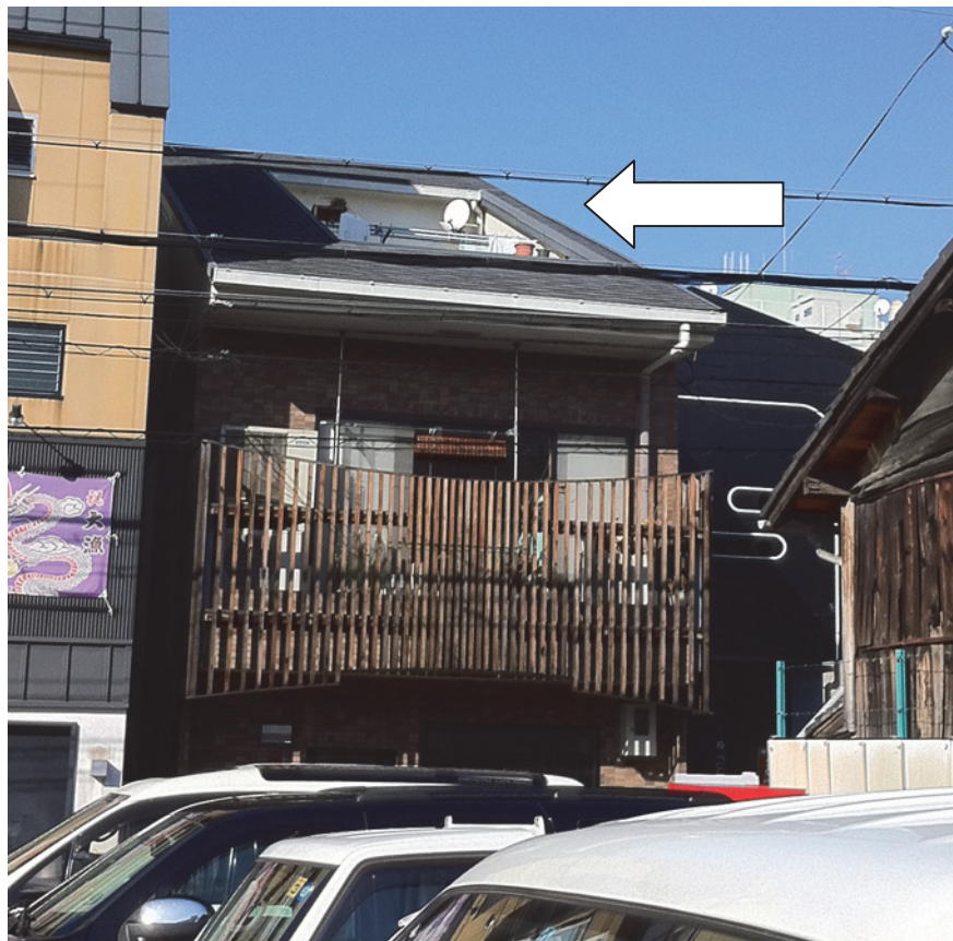
Fig. 7- 8 Roof terrace, which as well is used for clothes drying.
