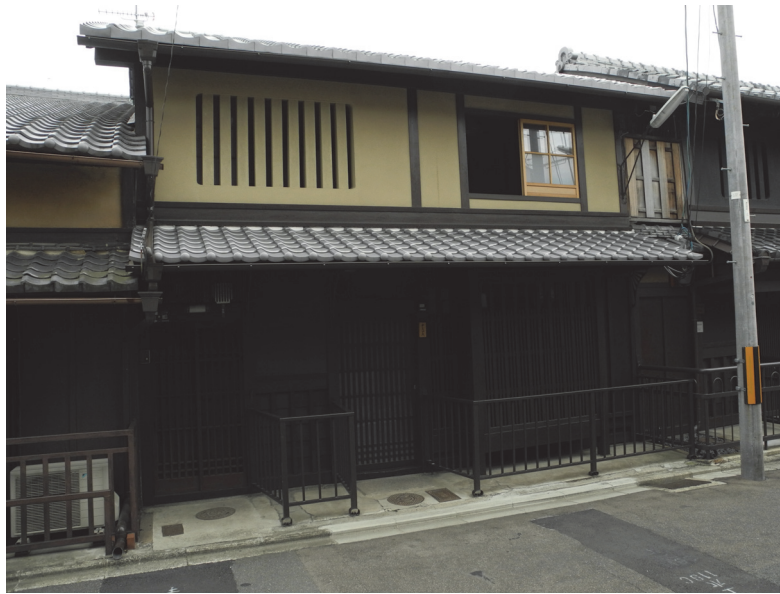
Fig. 6- 12 House corresponding to case 3 seen from the outside.
