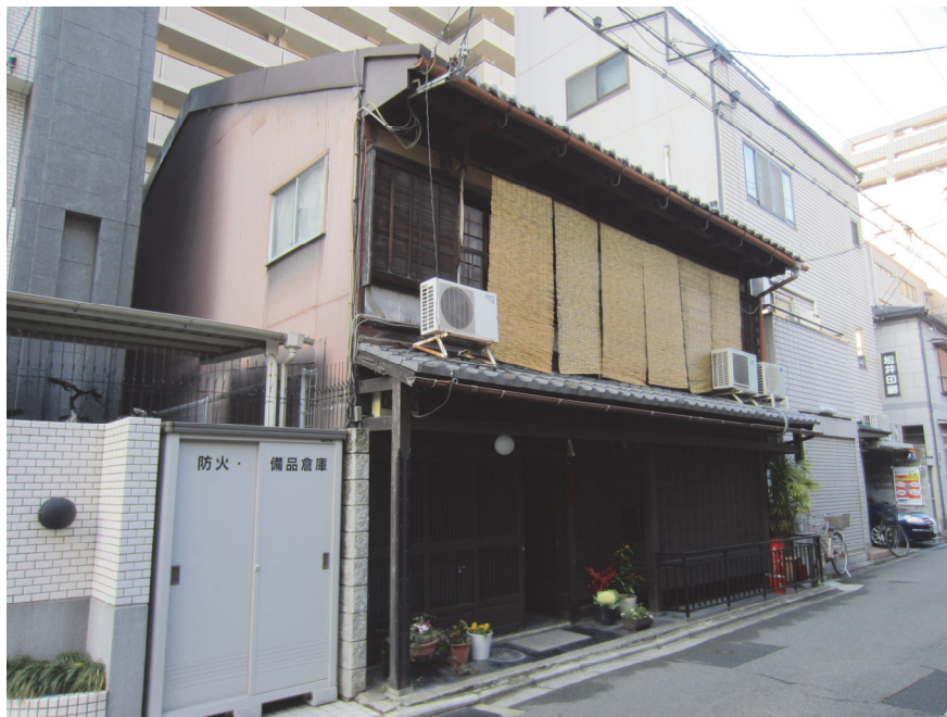
Fig. 6- 8 House corresponding to case 2 seen from the outside.
