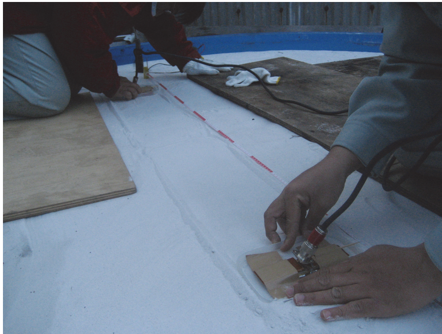
Fig.4.4-2 State of the efficiency test.
