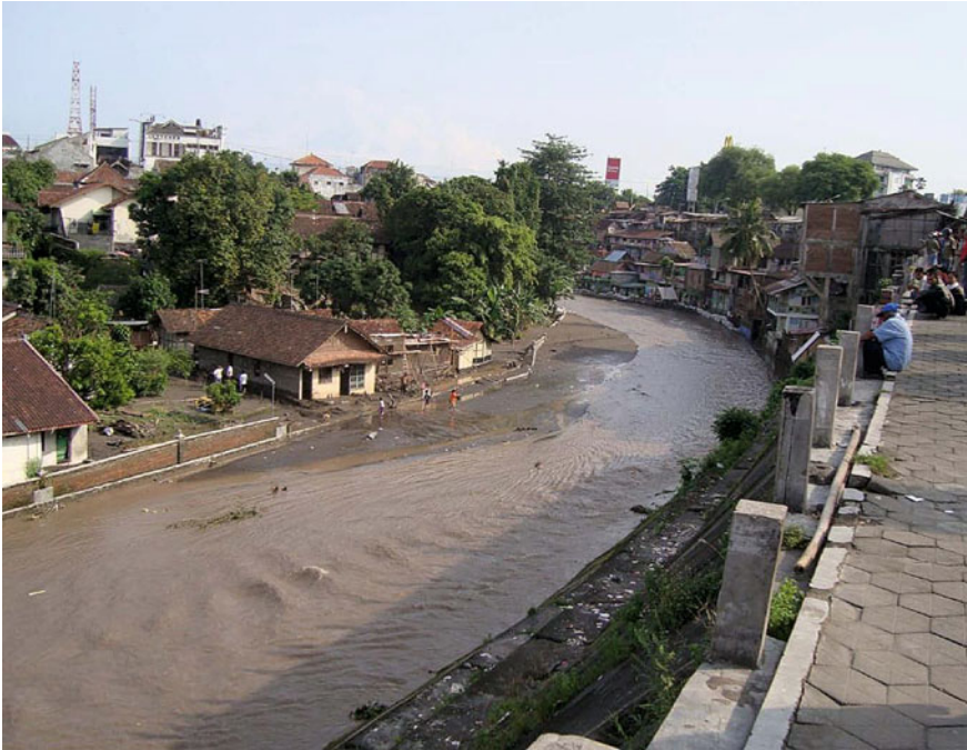
Fig. 6 Downstream condition of Code River: Jogoyudan area in the Yogyakarta City on 30 November 2010
