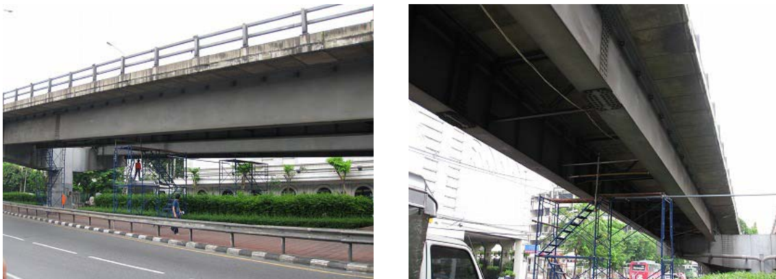
Fig. 5-3 Monitored bridge: two independent superstructures stay on common piers
