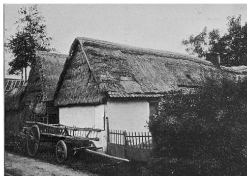
Fig. 7-2 Demangeon, 1907-House in the area of Prédefin, pointing out the materials of the construction thatch and slats
