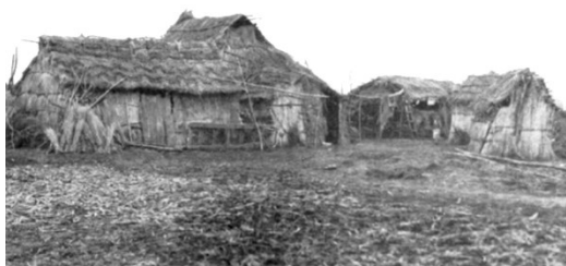
Fig. 7-10 Davis, 1934- Ainu house. Original caption: "The wall of rice straw (...) is designed to afford protection from cold winds"
