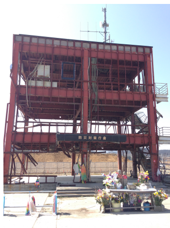
Figure 1.1: Steel-framed building in Minami-Sanriku, Miyagi Prefecture, Japan ravaged by the 2011 Tohoku-oki Earthquake Tsunami and left as a memorial
