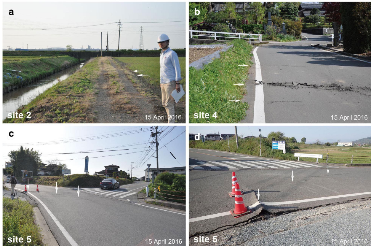
Fig. 3 Snapshots of surface ruptures related to the largest foreshock at each site shown in Fig. 1c and/or Fig. 2. a Small cracks on an unpaved road, indicated by white arrows. After the mainshock, two fault traces and a small depression between them were identified here, as shown in Fig. 4b. b Three rupture traces with right-lateral offset of a paved road. Total amount of offset was several centimeters. Five rupture traces were identified here after the mainshock, as shown in Fig. 4c, d. Total amount of offset was 13–14 cm after the mainshock. c, d Cracks on a paved road, indicated by white arrows. No lateral offset was recognized. However, a fault trace with right-lateral offset of ca. 30 cm was identified here after the mainshock, as shown in Fig. 4e–g
