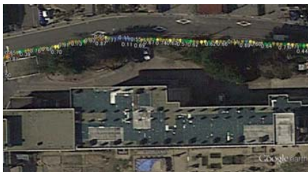
It's not possible to use high-pressure decontamination for high contaminated rubber sidewalks.
