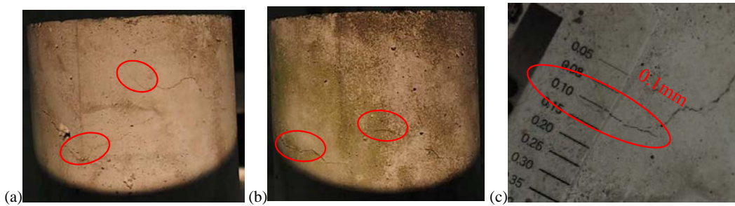
Fig. 3. Target cracks: (a) clean target surface; (b) dirty target surface; (c) closer look with a width gauge. (red circles mark the location of 0.1-mm cracks)
