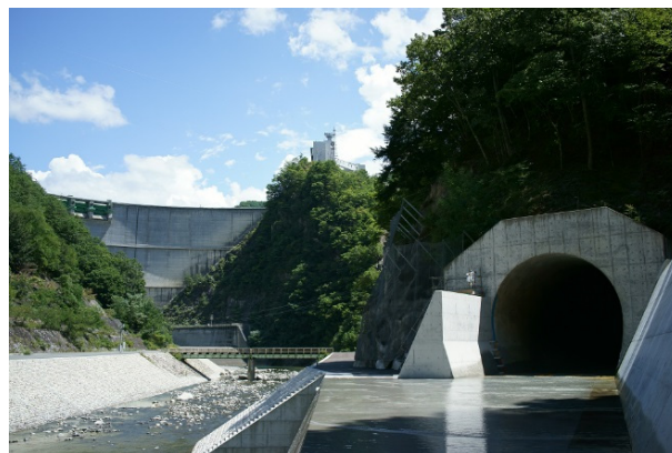
Figure 1: Outlet of the Koshiu dam SBT
