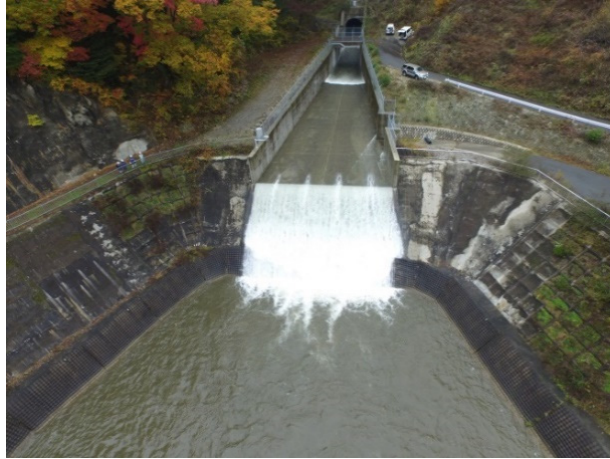
Fig. 12: Trial operation of sediment bypass (at the outlet)
