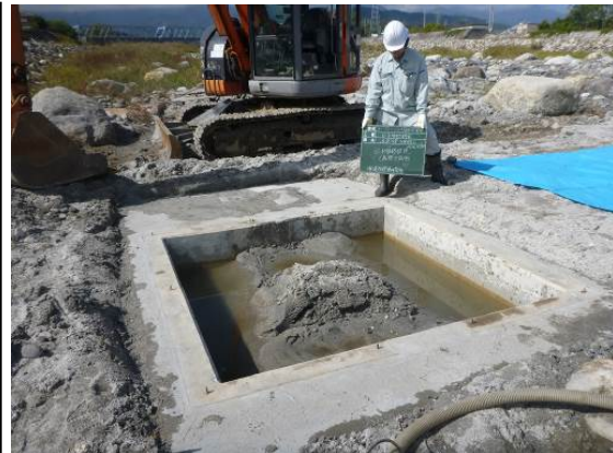
Photo 1: Sedimentation in the pit (2014 Typhoon No. 18)
