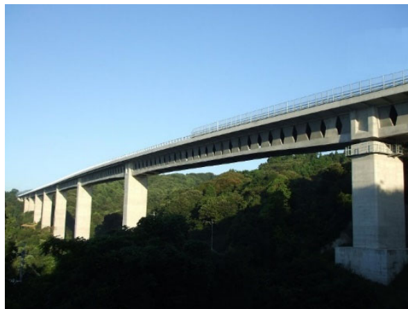
Fig. 1-1 Butterfly web girder (Takubogawa Bridge)
