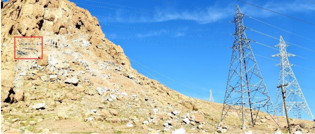
Fig. 1.5. Collapse of transmission tower due to rock fall on the mountains nearby the Sarpole-Zahab city.
