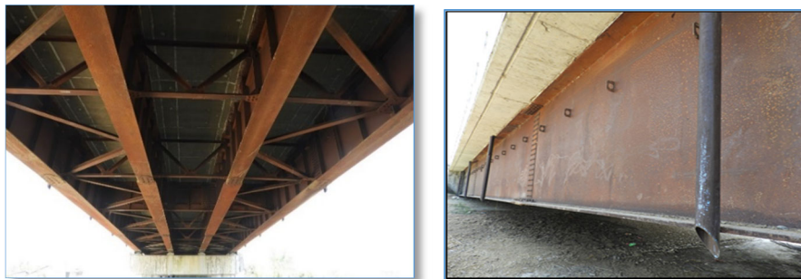
(a) Overall view of bridge underneath (b) Exterior girder
