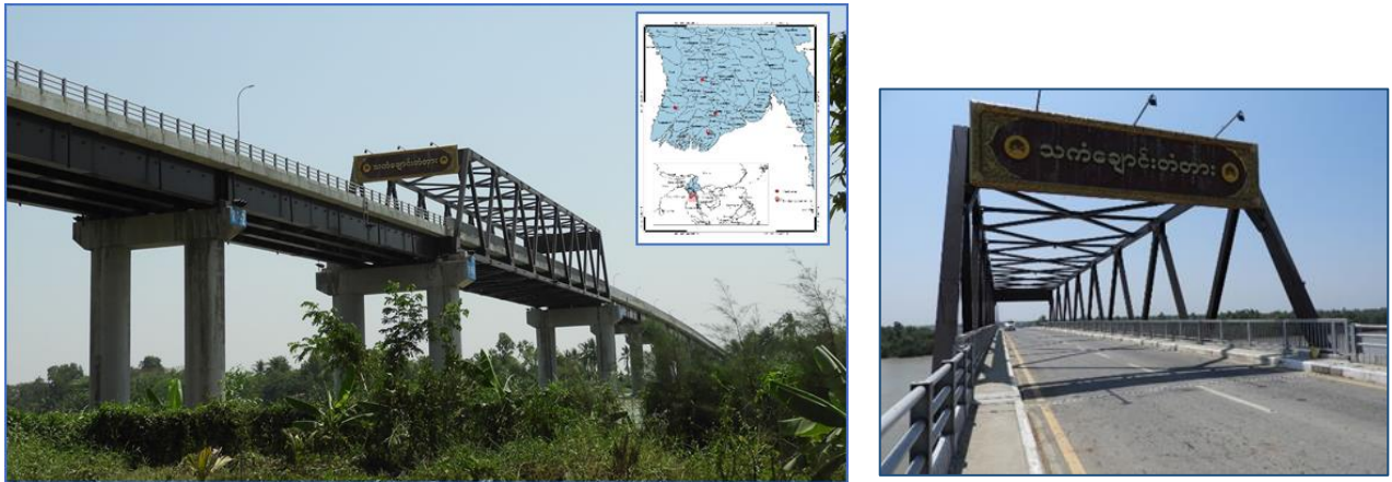
Figure 5.2 Thakan Chaung Bridge
