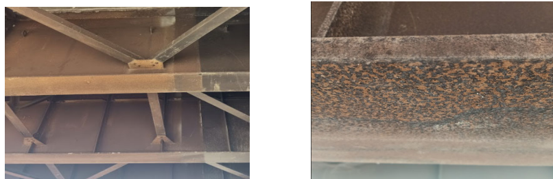
(a) Girder (close up) (b) Bottom flange (close up)
