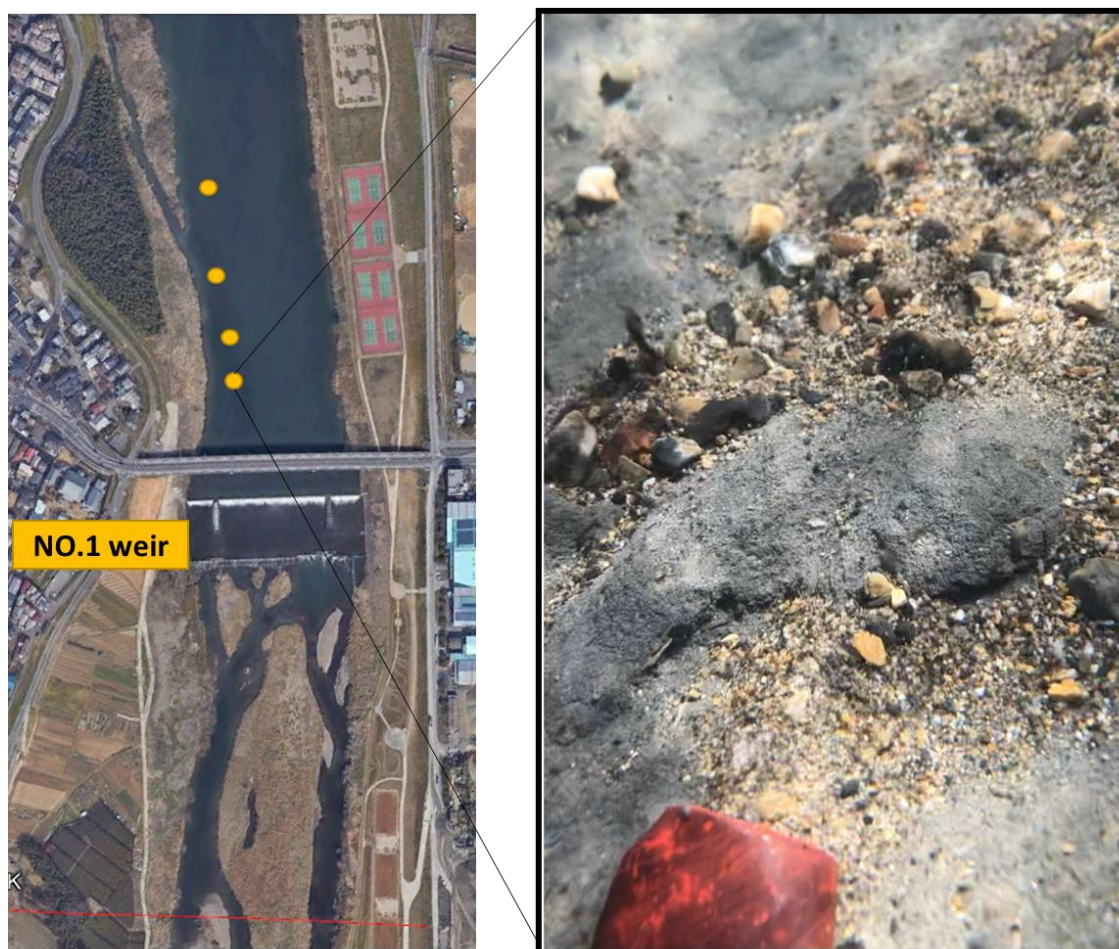
Fig. 5-27 Photo of riverbed surface upstream of No.1 weir during the removal.
