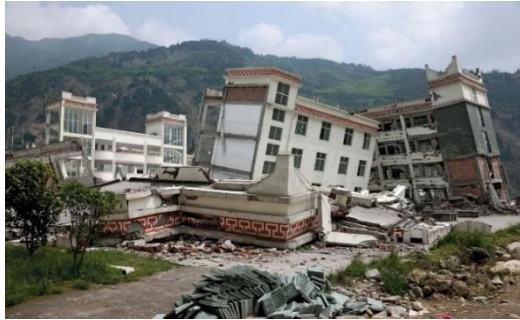
(a) School in Yingxiu, Sichuan province after 2008 Wenchuan earthquake (Kenneth Pletcher, 2008)
