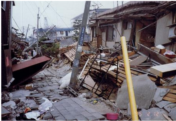
Photo 2 Total road blockage by collapsed wooden houses in Higashinada-Ward 3 weeks after the 1995 Hyogo-ken Nanbu (Kobe) earthquake (Photo by H. Kawase).
