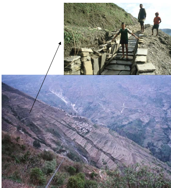
Fig. 21 A settlement threatened by gully erosion and their own countermeasure facility.
