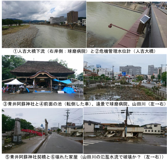
Fig.4 Flood damages in Hitoyoshi city area
