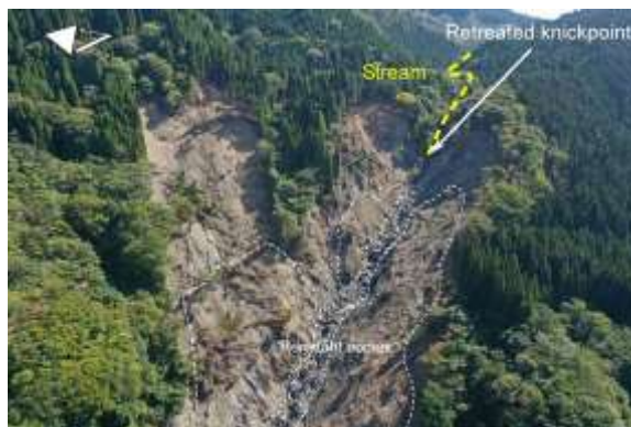
Fig. 8 The overview of Gumeki Valley landslide and geomorphological explanations.
