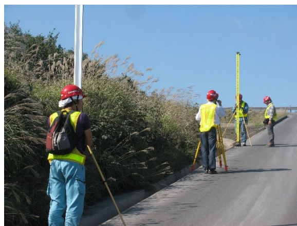
Photo 1 Basic members during leveling survey
