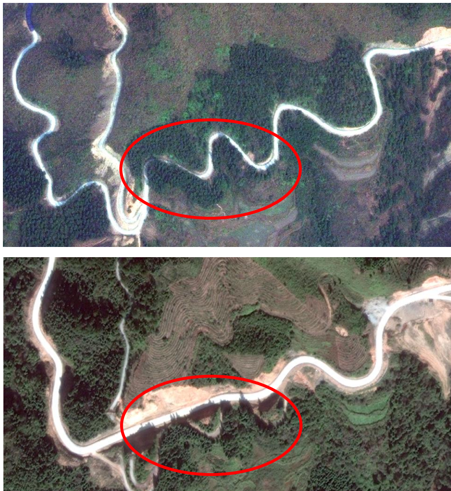
Figure 4.14. Road construction that caused fragmentation in Gaoyou village. (upper: 2009, lower: 2020)
