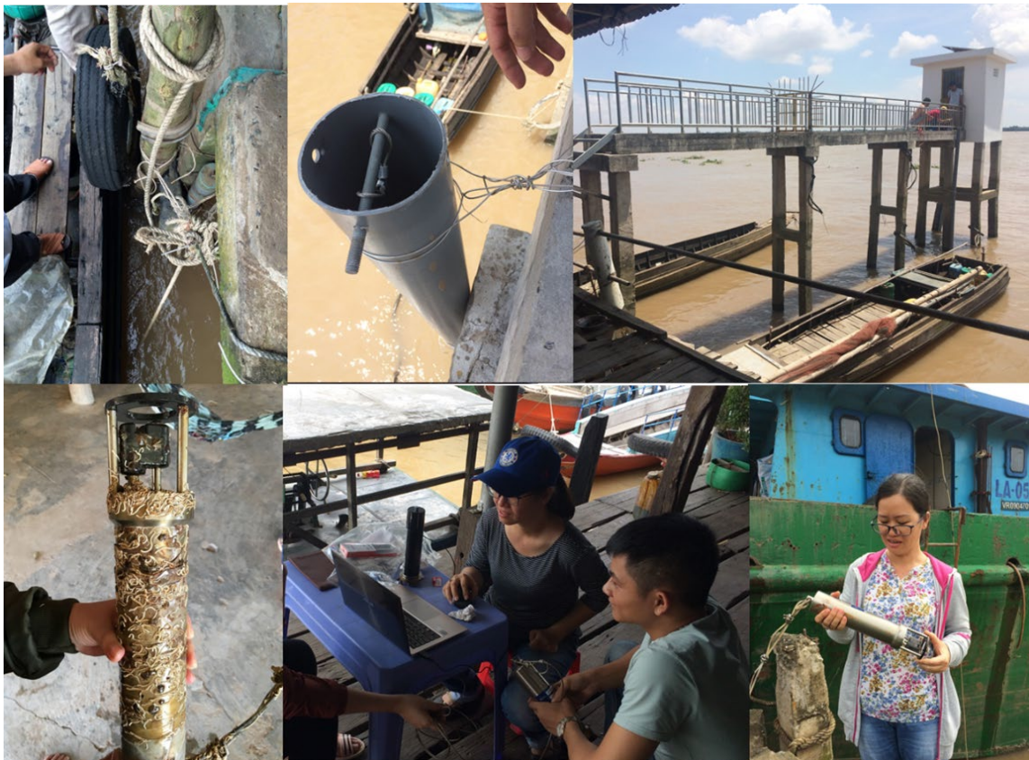
Figure 3.5 Field activities in installing salinity stations
