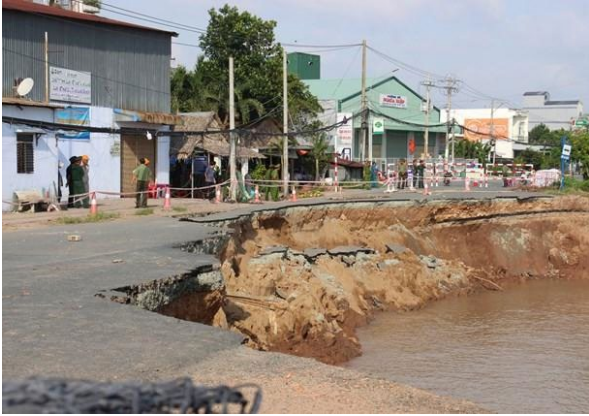
Figure 5.1 On 1 st August 2019 at AnGiang, the bank erosion is 80m long and 25 wide.
