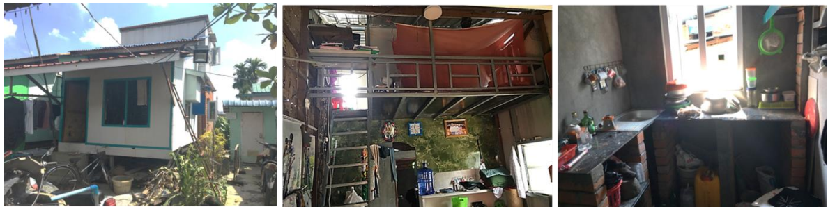
Figure 5.8 Exterior and interior of House 18
