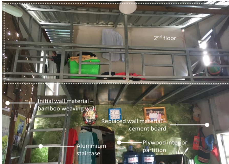
Figure 5.9 Interior of modified two-storeyed house (House 18, Site 1)
