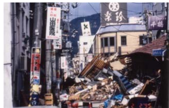
Photo 5. Collapsed houses near the Sannomiya Station, Kobe (taken on February 2, 1995, by M. Hashimoto).
