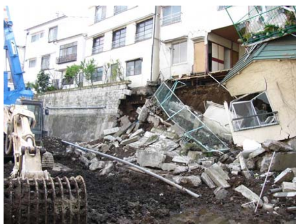
Photo 3 Collapse of small residential fill in Tokyo, 2004
