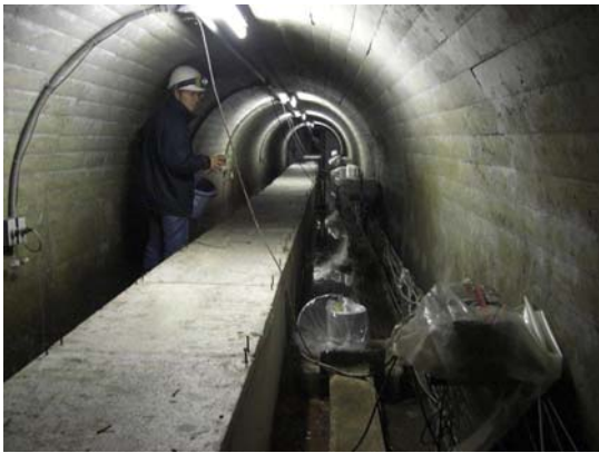
Photo 4 A seismometer installed in the Yasutomi observation tunnel of the Yamasaki fault
