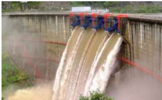
Photo 5 Outflow from the crest gates of the Yahagi dam
