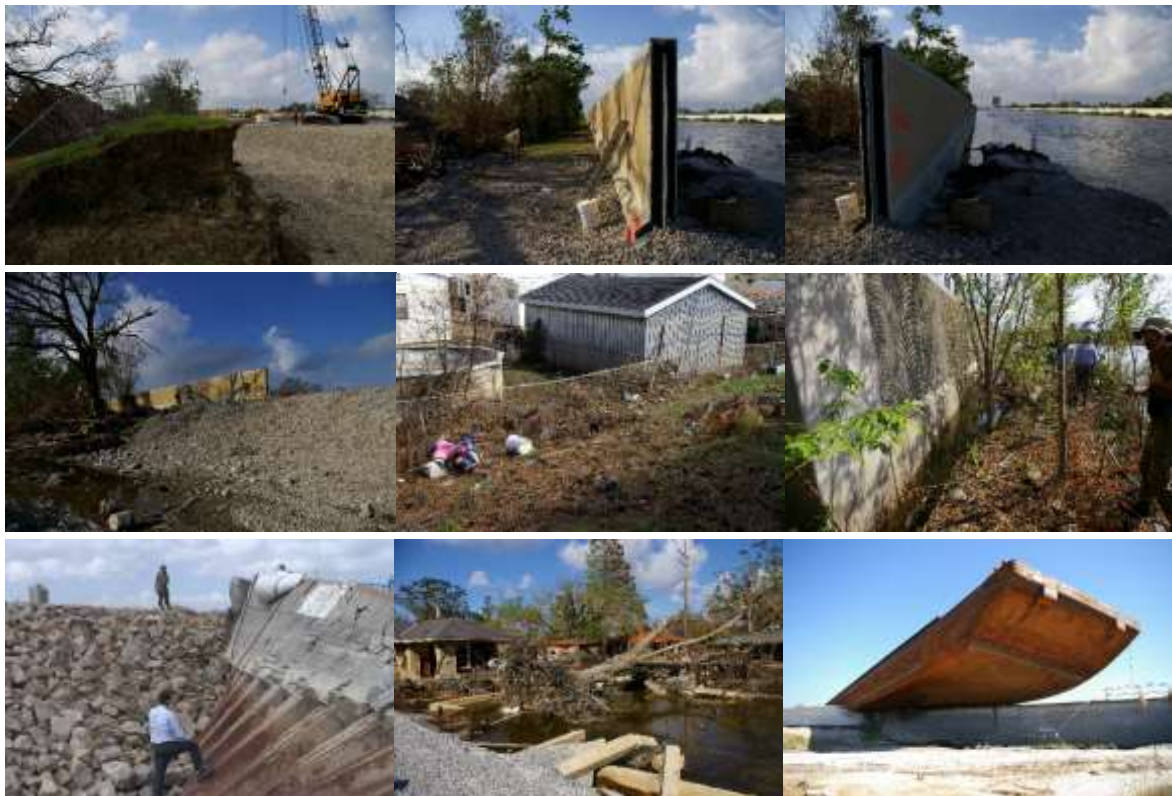
Photo 8 Hurricane Katrina's damages of storm surge protection levee system in New Orleans.
