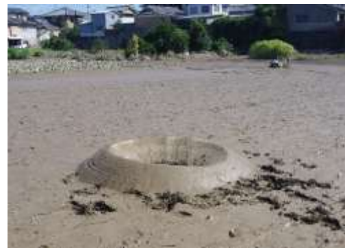
Photo 11 Sand boiling at the farmland beyond the left embankment.
