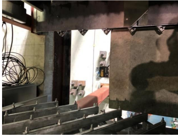
Figure 6-3 EXP.J at the connecting bridge
