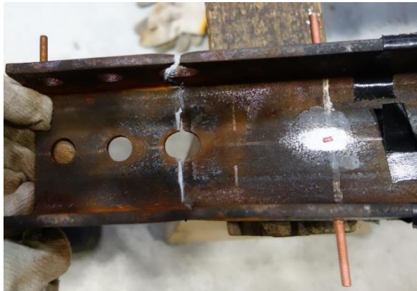
Figure 2-26 Fracture of IHCB-F40W60 at the brace end
