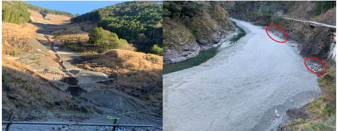
Figure 3-3 The sediment sources upstream of Otsutachi dam. Left figure: The landslide of the mountain. Right figure: The sediment for replenishment including classification.
