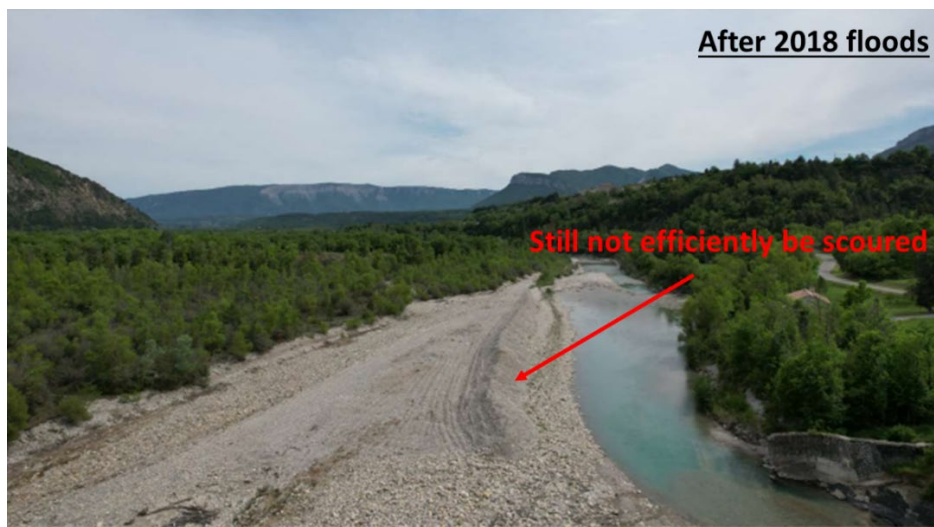
Figure 4-36 The remaining sediment at the replenishment site after the 2018 SR in the Buëch River.
