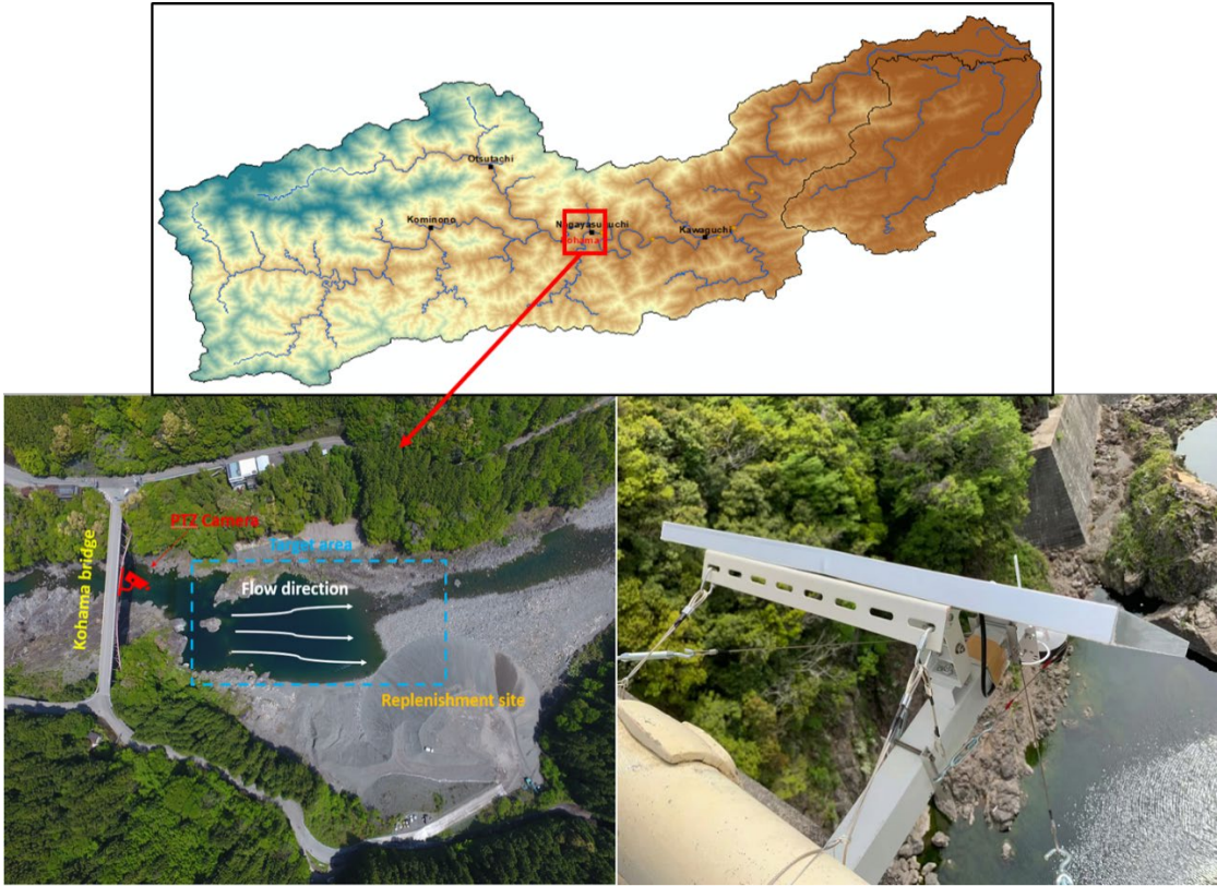
Figure 3-25 The location of camera installed on the Kohama bridge. The left figure shows the plan view of the camera location and replenishment site. The right figure shows the PTZ camera with solar panel.
