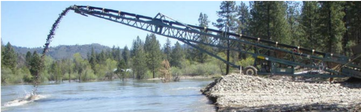
Figure 2-7 High-flow injection as the replenishment approach implemented in the Trinity River (Krause, 2012).
