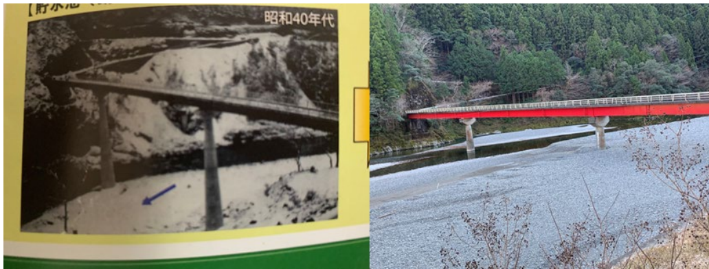
Figure 3-5 The potential sediment sources upstream of Kominono dam shows significant bed aggradation. Left figure: Photo in 1965 (from the report of Naka River). Right figure: Photo in 2020.
