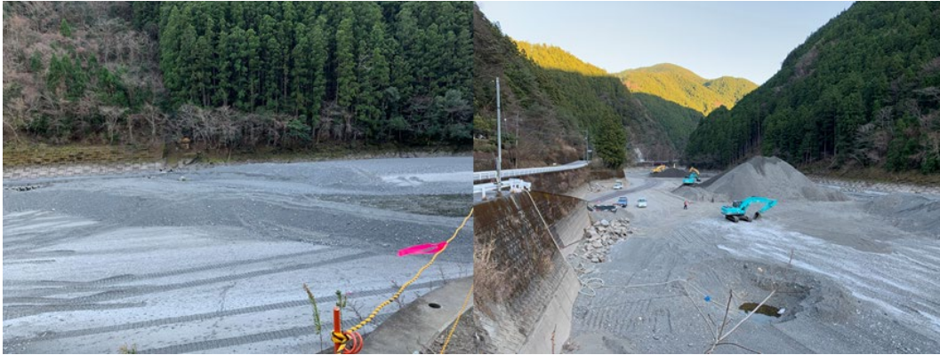
Figure 3-4 The sediment excavation downstream of Otsutachi dam.
