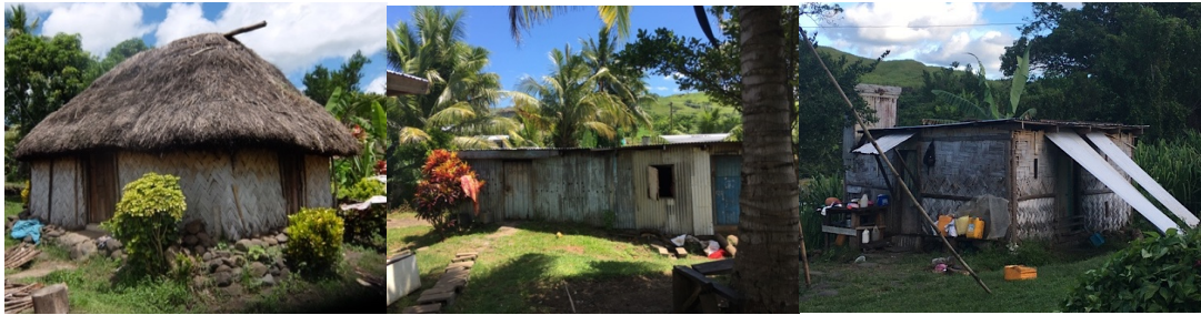
Figure 5. 10 Traditional house ( bure ); (left) modern house made of corrugated iron sheets (middle) mixed housing structure with bamboo walls, timber structure and CI roof (right) (Source: Mari Miyaji)
