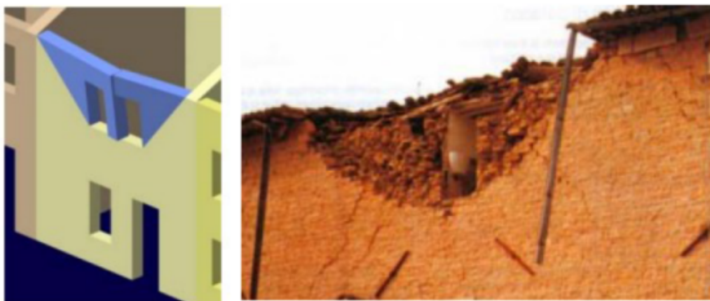
Figure 6: The horizontal arch mechanism in masonry façades [13].
