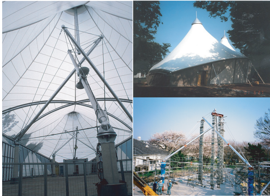
Figure 1.6: Example of a pair of tensegrity structures used as frames to support a membrane roof, constructed at Chiba in Japan in 2001. (Architectural design by A. Fujii and structural design by K. Kawaguchi.) The left photo is the interior view of the building, the upper-right photo is its exterior view and the lower right is one of the tensegrity structure under construction. The photos are kindly provided by one of the designer, Professor K. Kawaguchi at the University of Tokyo.
