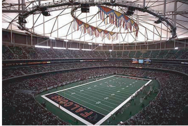
Figure 1.5: Inside view of the Georgia Dome, a special tensegrity structure. It was built in Atlanta U.S. in 1992 for the Atlanta Summer Olympic Games. It is a multi-purpose public stadium, that can be used for American football, concert, basketball and gymnastics.
